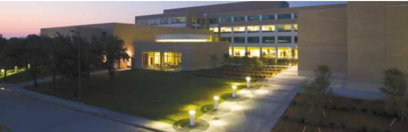
The Drive A side of the building at dawn
